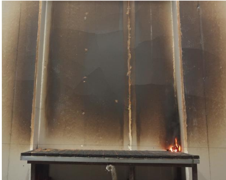
Fig. 3 Exposed Side after the radiant heat test
